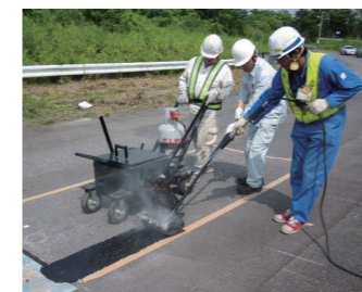
段差補修・亀の子ひび割れ補修
